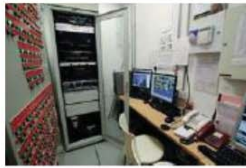
Inside the control room
