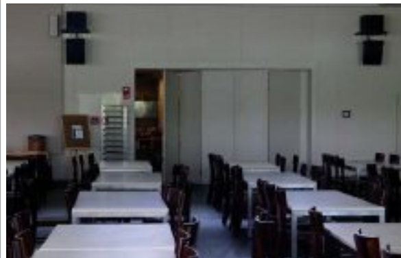
A cafeteria with a TOA HX-5 line array requires Nion NX processing
